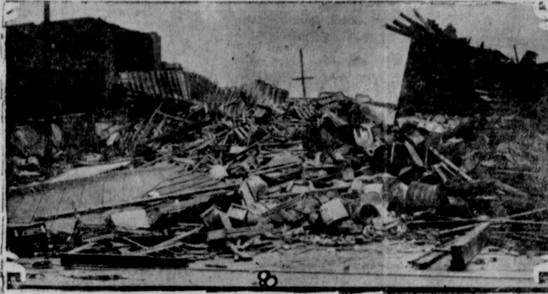
During a storm which swept from Illinois to Pennsylvania, the five-story brick building occupied by the Isaac Walker Hardware Company at Peoria, Ill., collapsed. Two men were killed when the building crushed a two-story garage next door.
