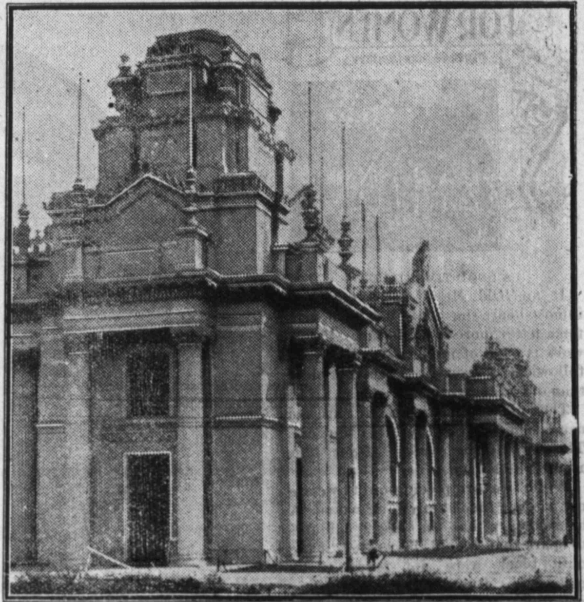
A CORNER OF PALACE OF ELECTRICITY, WORLD'S FAIR, ST. LOUIS.
