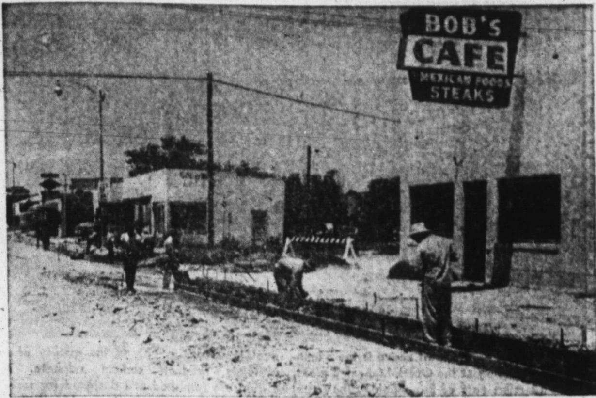
SETTING CURB FORMS — Construction on forms for curbing along the right-of-way. Most Lubbock Road took another step toward curbing was completed or had forms ready for completion this week as workmen began setting completion by mid-week. (Staff Photo)
