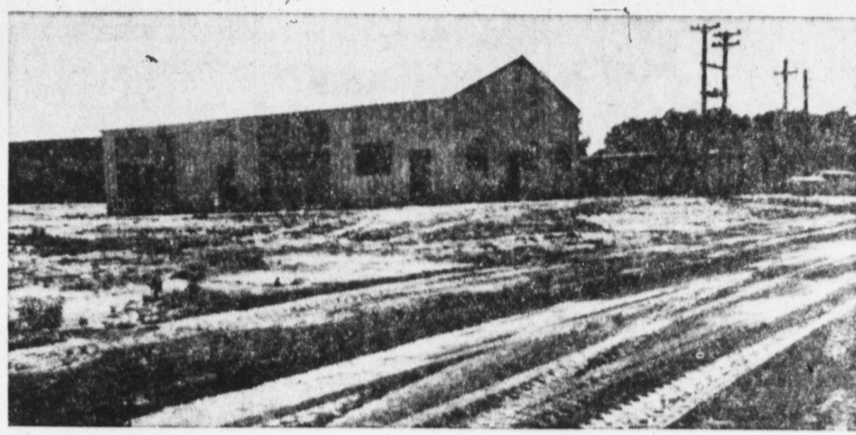
WATER FOCAL POINT —City water department activities will be centralized in this area when construction is completed this month. Building in foreground will house maintenance shop and offices. The building at right is recently completed pumping station and the structure at left is a portion of the one million gallon water storage tank. (NEWSfoto)
