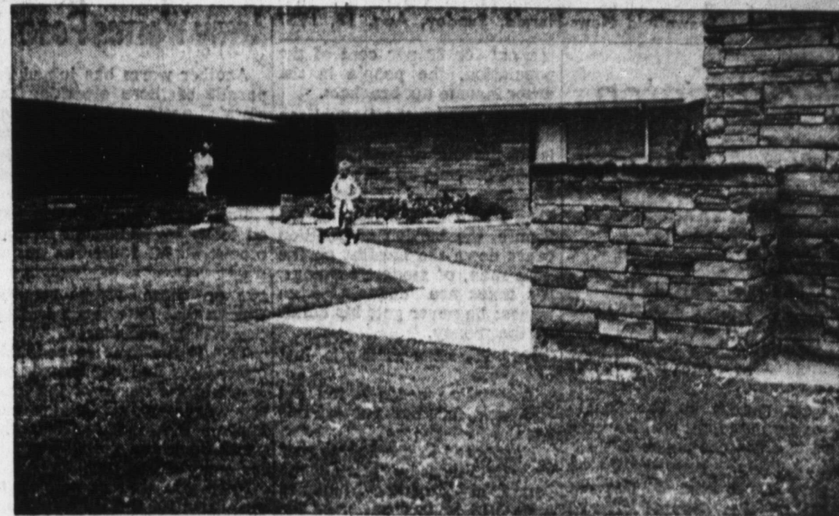
BACKYARD FUN — is enjoyed the year round in this handsome setting. The low stone banister encloses a curved patio off the den. The roof of the patio is of corrugated plastic that provides ample shield from the sun, yet lets all the light through. The barbecue pit in the foreground is used often and the walk leading from it to the patio makes a fine highway for Duane and his tricycle. (NEWSfoto)
