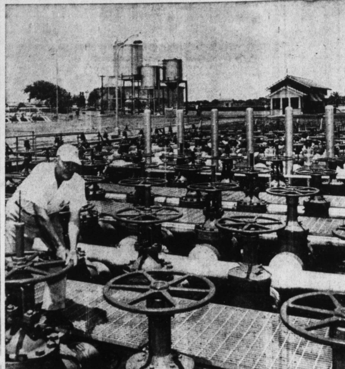
STEERING WHEEL — An employee of Humble Pipe Line Company at Webster Station turns the right "steering wheel" to direct a stream of oil to its proper destination. Crude from one of Websters 49 storage tanks before being dispatched to a manufacturing or shipping point. Pumps at Webster can move as much as 185,000 barrels of oil daily.
