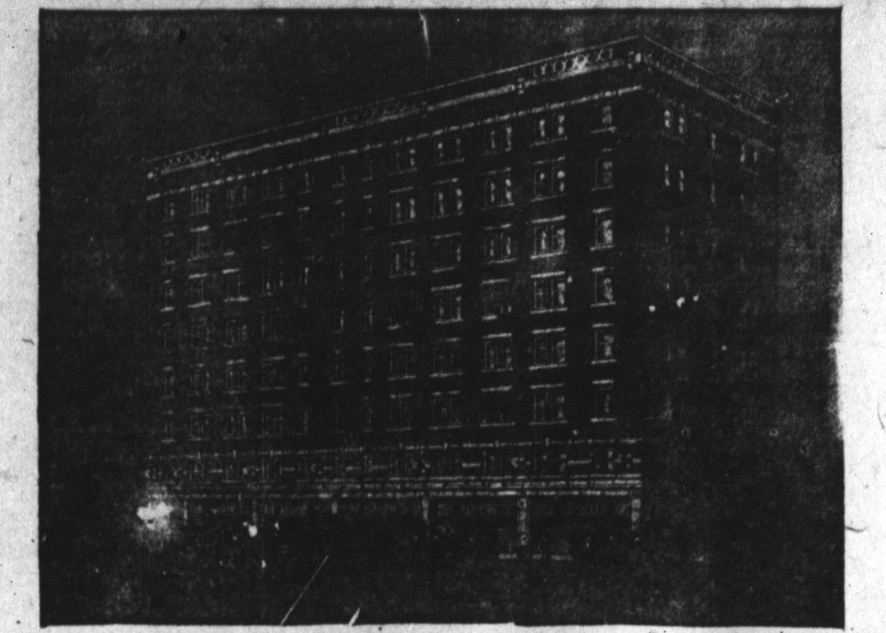
The eight story office building being erected by the Amarillo Building company at Third and Folk streets, Amarillo, here shown, starts a building program which promises to be a forerunner of great events for the Queen City of the Plains.
