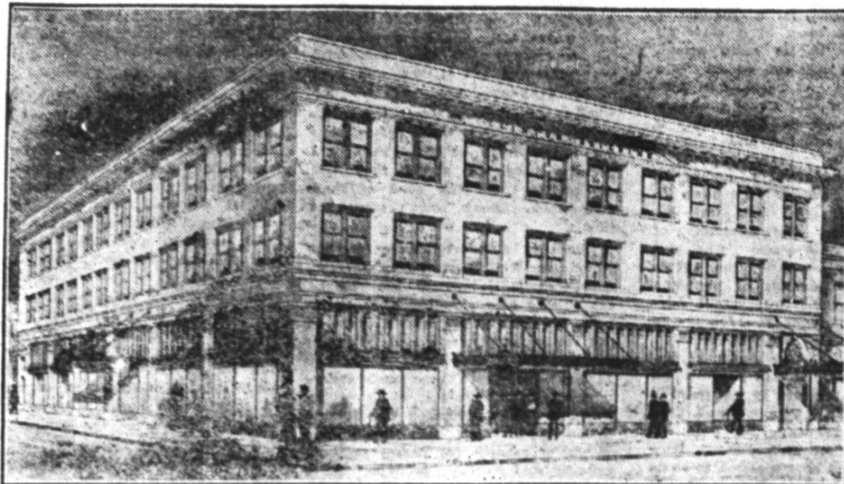
Clinton Building, Third and Chestnut Streets. Under Construction
