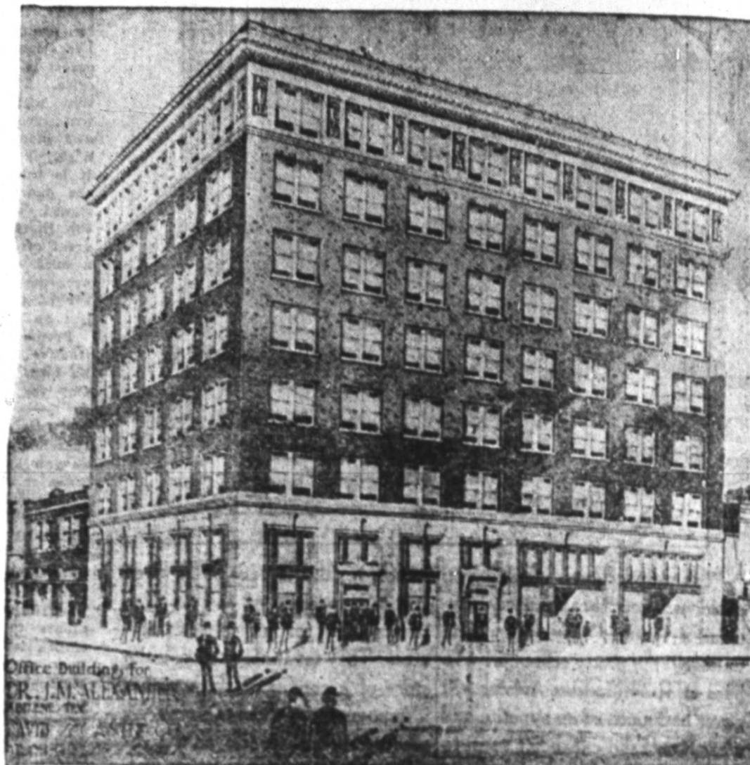
Alexander Building, North First and Pine. Exterior work Complete
