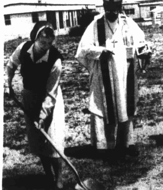
GROUNDBREAKING — Sister Lucy Keane turns a shovelfull of dirt to break ground for the Immaculate Heart of Mary School's $100,000 science laboratory and learning resource center Friday. Bishop Joseph Anthony Florenza, bishop of the Catholic Diocese of San Angelo, looks on. Bishop Florenza celebrated a "Mass of Thanksgiving" to provide an auspicious beginning for the new addition, which is expected to be completed by the beginning of the 1982-83 school year.
