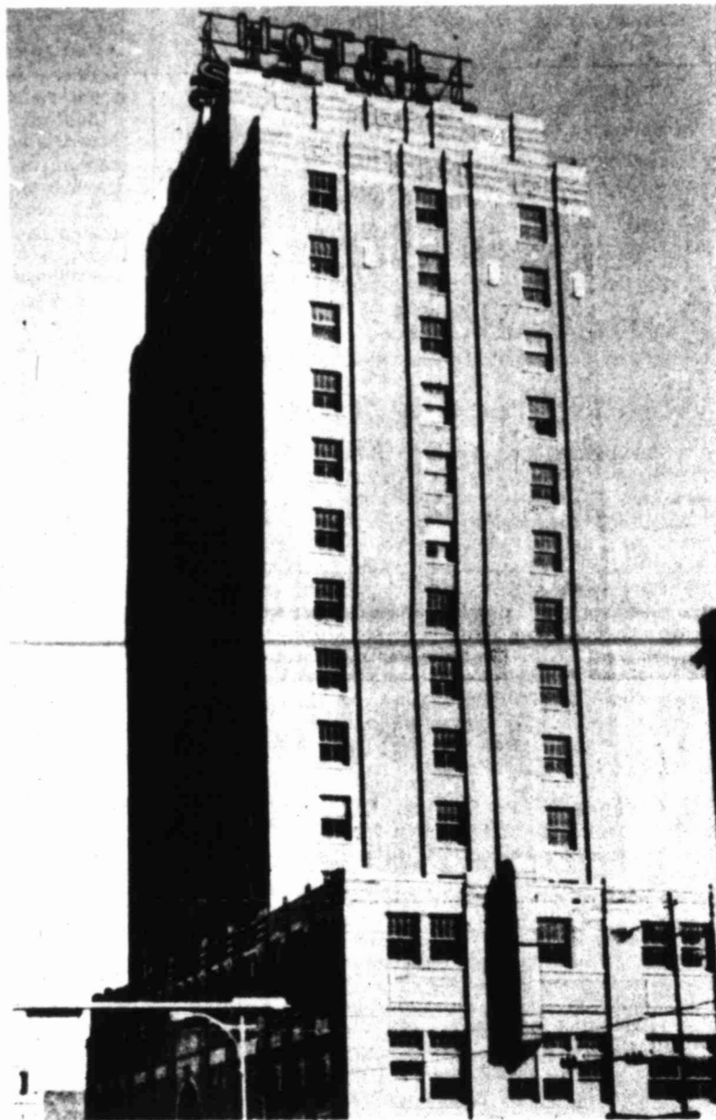
HOPE FOR THE HOTEL — Dallas entrepreneur Robert Kendall says $4½ million and his expertise can restore the Settles Hotel to its original 1930s condition. The problem is finding investors interested in the project, he says.
