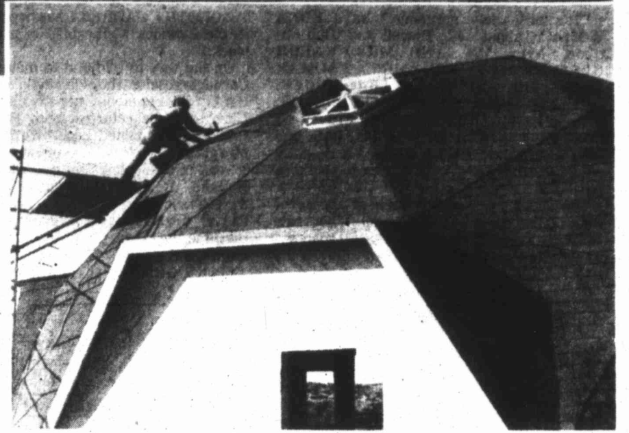
SHINGLING THE ROOF — Jimmy Hopper shingled the top of the roof of his geodesic home by tying a rope to himself on one side of the house and to a skylight on the other side. A scaffold was used to shingle the lower part of the roof.
