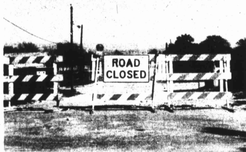
ROAD CLOSED — Street barricades block traffic from entering Goliad Street which is under construction in a street improvements project behind schedule.
