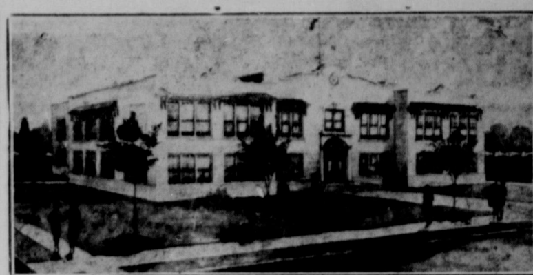
Friona grade school. This is a splendid, modern brick building housing the lower grades. Pupils are brought to Friona school from as far as twenty miles in modern busses operated for their convenience.
