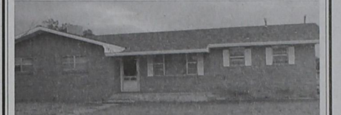
3/2 Brick with carport on large corner lot $58,500
