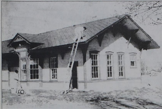
IN 1988--Work continued on the exterior renovation of the Depot building.
