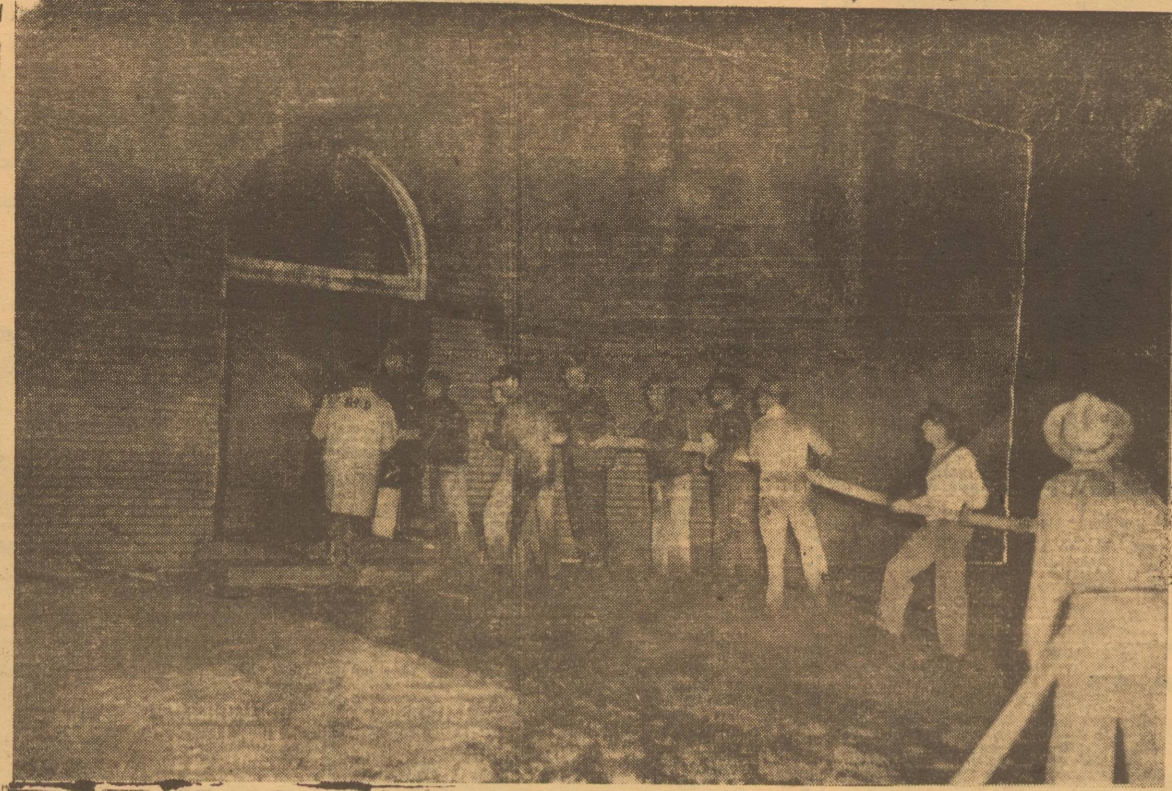
Shown here are Friona and Hereford firemen battling the blaze at the fire which last week demolished the high school auditorium here. Frionans on this hose have been identified as John Gaede, Troy Kemp, Bill Smith, Raymond Jones, and Roy Hollis.
