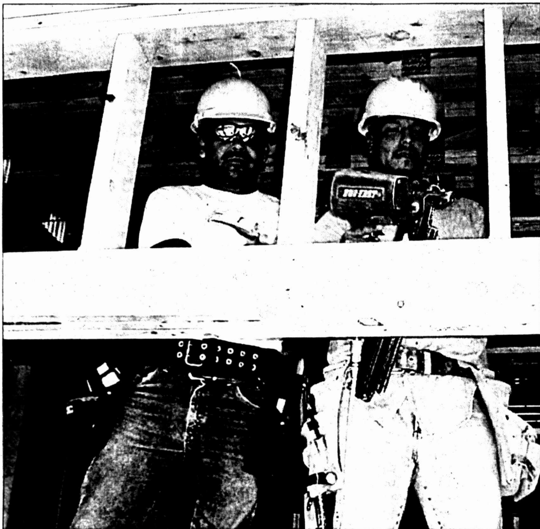
Juan C. Moreno, left, and Daniel Delgadillo, workers with RM Construction of Abilene, are part of the crew building the Holiday Inn Express at the intersection of Interstate 20 and Highway 87. The hotel is scheduled for completion in mid-October.
