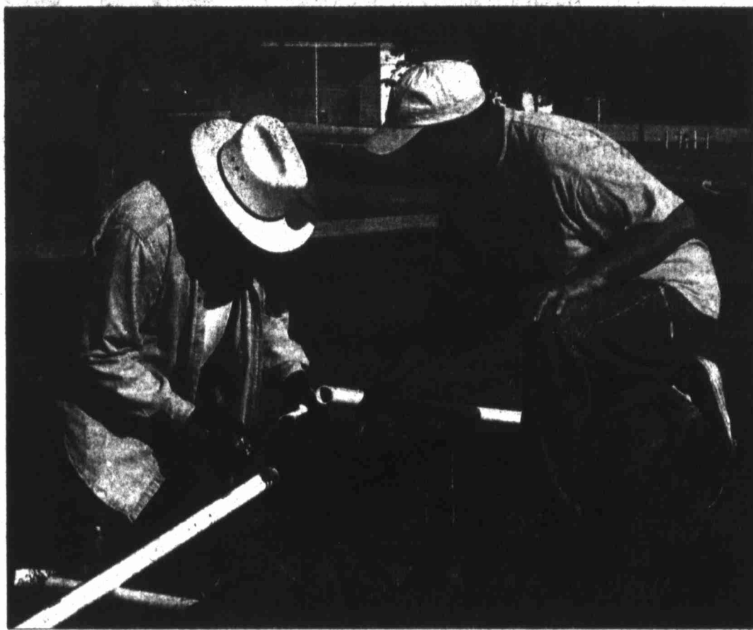
Wayne Stroup, left, and John Ybarra help install an irrigation line at the Spring City Senior Citizen's Center Thursday morning. Members of Leadership Big Spring installed the lines as part of the group's annual community service project.
