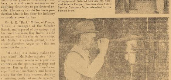
This heavy duty electric drill and drill press, plus a good supply of hand tools, plus a good mechanic all add up to make this shop a "money maker". Ray Roles, the ranch foreman, is operating the electric drill.
