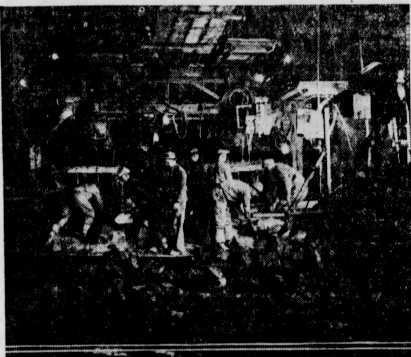
Here is a scene 30 feet below the bottom of the Hudson river, and 170 feet out from the Weehawken shore line, as engineers and sand hogs, working under 13 pounds of air pressure, thrust the giant tunnel toward Manhattan, at a rate of 30 inches at a time. This tunnel is meant for interstate motor traffic.
