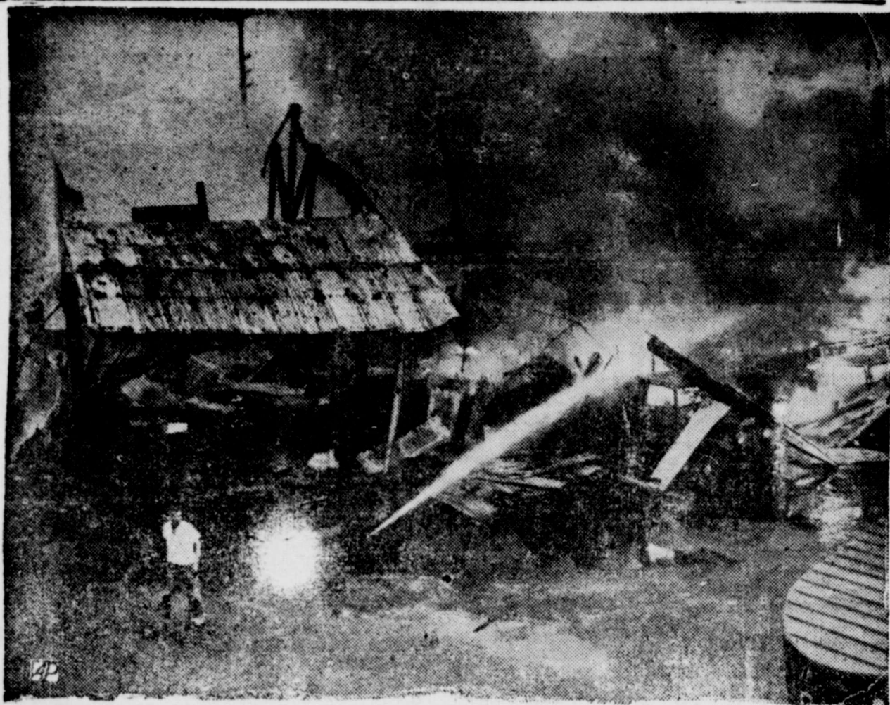
RAIL WRECK NEAR REFUGIO Fireman O. R. Workman of Houston, was killed when this
