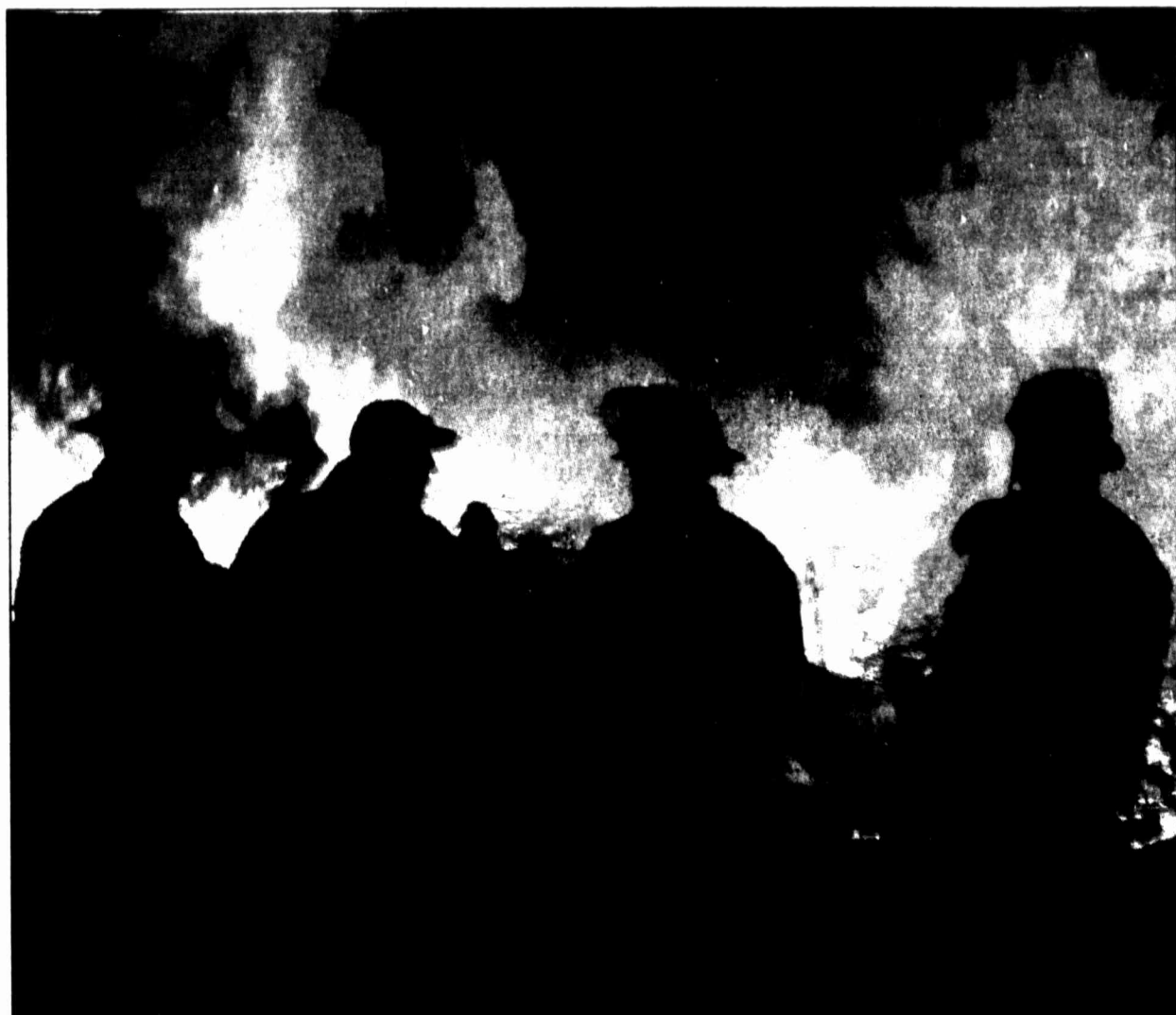
Four Howard County Volunteer Fire Department personnel are silhouetted against a bonfire organized by the Coahoma community development group Saturday evening. The bonfire contained the remains of four dilapidated structures demolished during a community wide cleanup effort last December.
