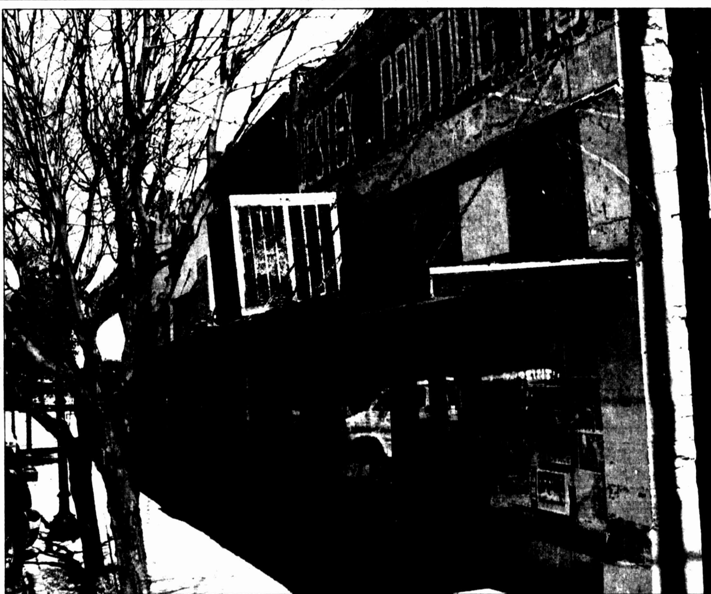
These shops will be among the 17 buildings targeted for renovation in the Heritage Square project, an $8 million downtown revitalization plan that encompasses 300,000 square feet.
