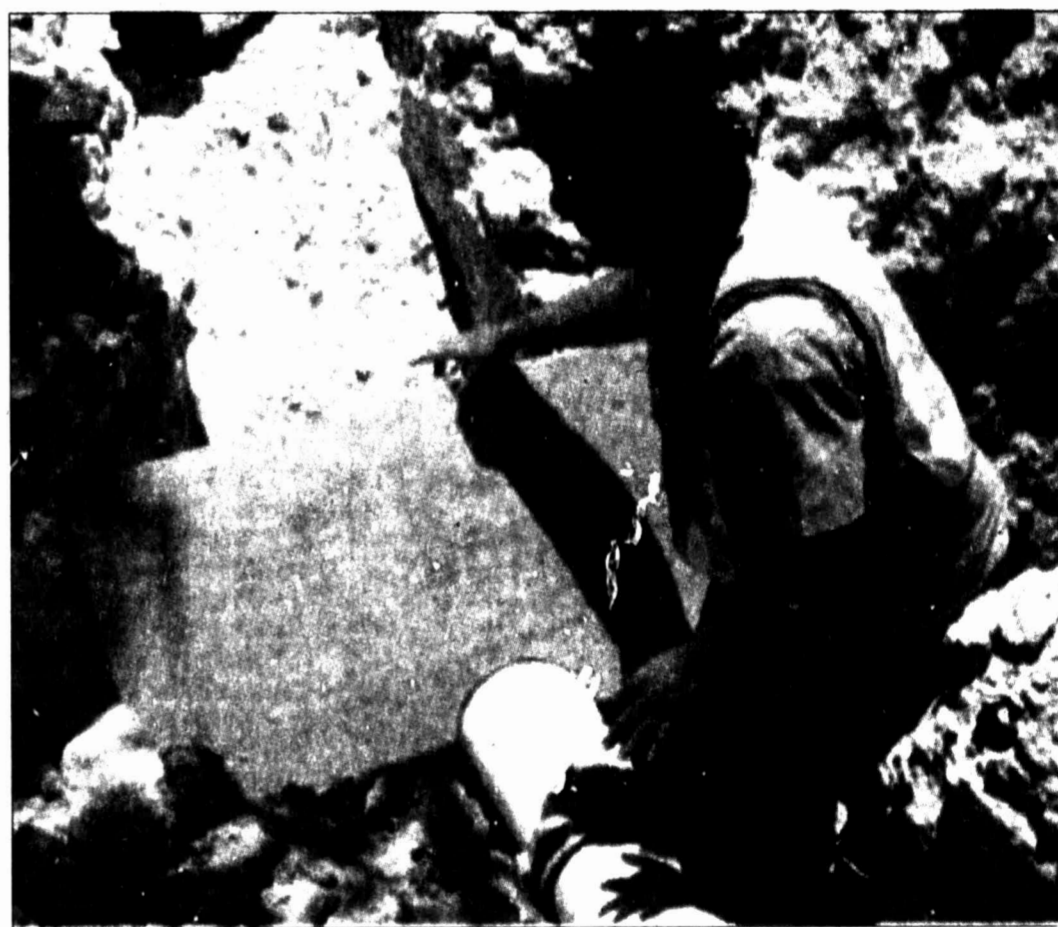
HERALD photo/Thomas Jenkins Steve Salinas, a crew leader with the city of Big Spring water department, prepares a water line to be encased in concrete near the intersection of 24th Street and Main. Part of the city's water line replacement project, the crew is replacing all of the main water lines on the block.
