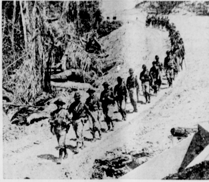
Men of the 14th Infantry hike along the clearing of the new trans-isthmian highway in Panama as they cross the isthmus for maneuvers. With the defense highway scheduled for completion this year, army officials believe this will be the last time that mobile force soldiers will have to make the trans-isthmus crossing on foot.
