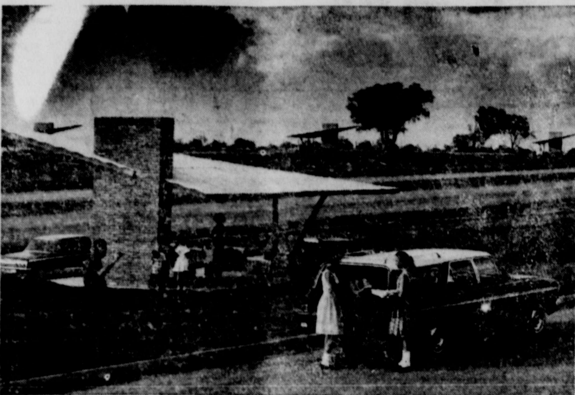
The Interstate Highway System in Texas is being blessed with large, elaborate Safety Rest Areas for the safety and convenience of Texas travelers. Motorists can now relax and refresh themselves in the first of these rest areas (roadside parks) designed and built on the Interstate Highway System in Texas. This new rest area contains eight arbors equipped with fire places for family cooking, incinerators, fire wood, and big spacious tables and benches for picnicking. The "park" lies on a small knoll ten miles east of San Antonio on Interstate Highway 10 and was formally dedicated May 29.
