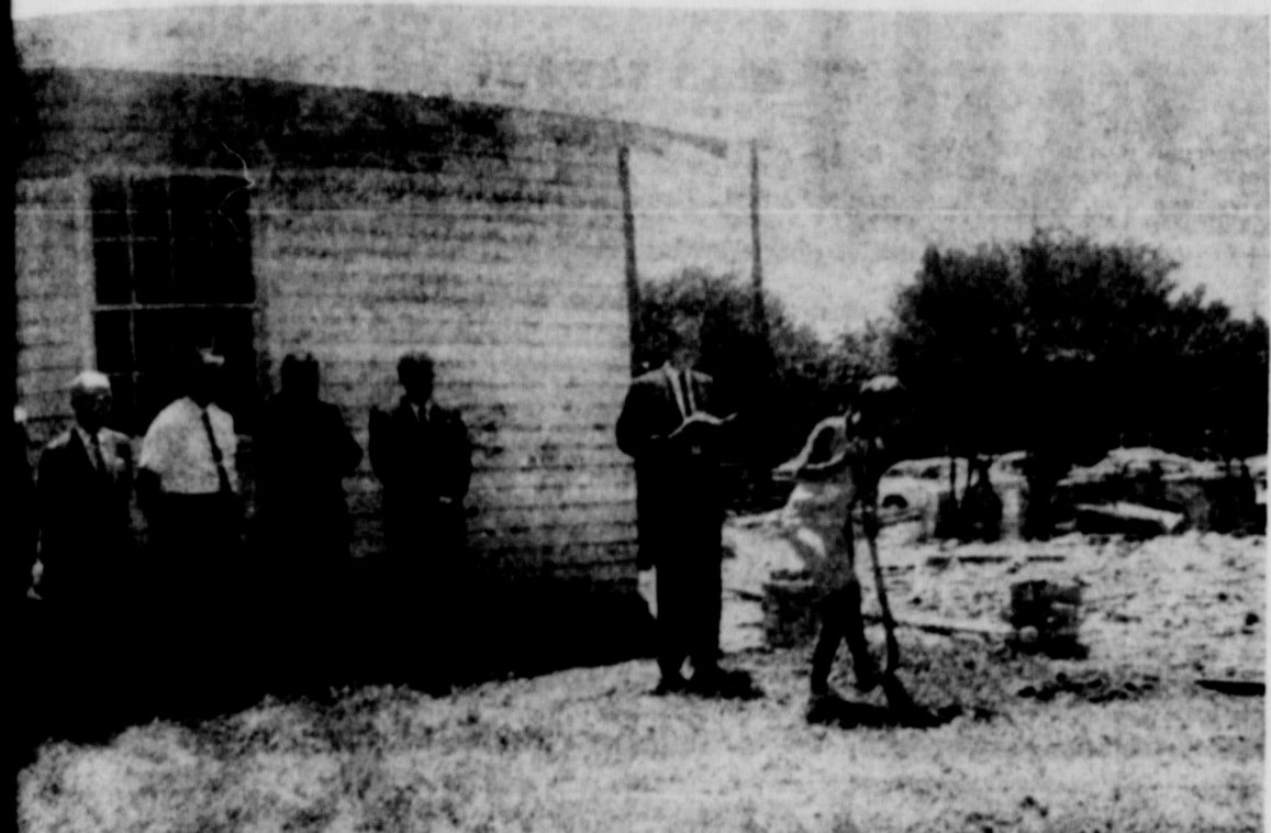
FIRST BAPTIST CHURCH members participated in ground-breaking ceremonies Sunday in preparation for construction of their new building. Shown here are Jane Akin, representing the Youth Council, as she turns a spadeful of earth. Others in photo, from left to right,
