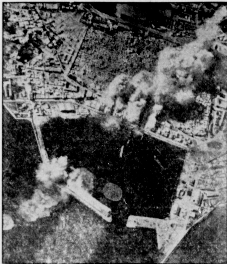
Direct hits on harbor warehouses, terminals and a pierhead at Sousse, Tunisia, are scored by U. S. Army Air Force bombers as part of the program to smash axis lifelines by destroying supplies.
