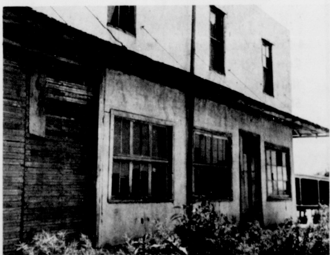
GARDEN SPOT? . . . Friona, which once had the title "Brightest Spot on the Golden Spread," has some scenes on the highway and elsewhere that makes one wonder if it can still live up to the title. The above photo, of an empty building on the south side of Highway 60, is one of the sights which greets people as they enter the city. (See letter, comments in "Star Lives" column)
