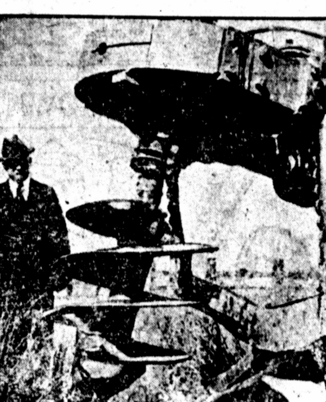
This huge boring machine plants telephone poles a day. The auger digs a hole seven feet deep and two feet in diameter. The machine then lifts a 60-foot pole and sticks it in the hole. Three minutes to a pole.
