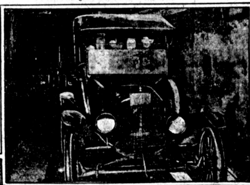
One of the procession of cars circling through the elliptical tunnel. Note the air duct boxes beneath and overhead.
