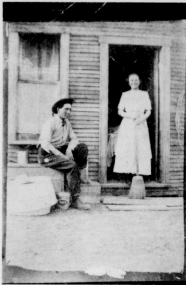
OUR FIRST HOME. . . Mr. and Mrs. Floyd Schlenker are pictured here soon after their first home was completed in 1913. A few years later the couple sold the New Mexico claim on which this house was located and moved the house over into Parmer County, where it formed a part of their first Texas home.
