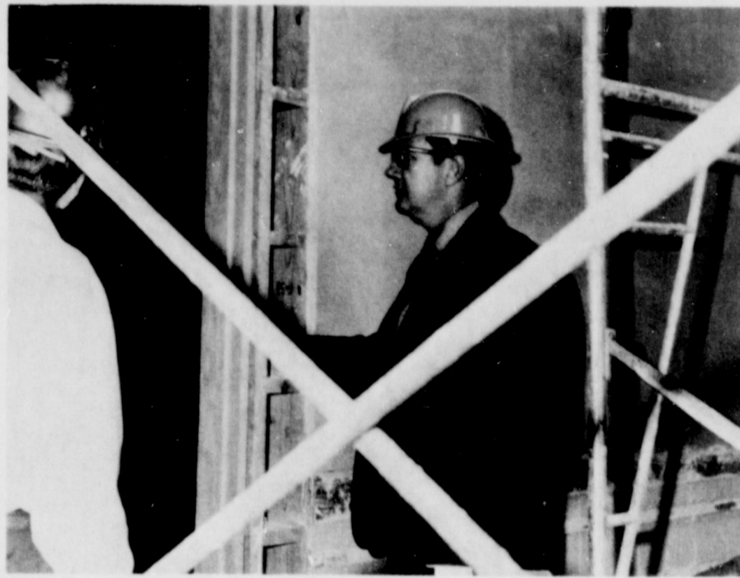
SENATOR JACK HIGHTOWER, Chairman of the Senate Contingent Expense Committee, supervises part of the work project being undertaken at the State Capitol. Senator Hightower is wearing a new "hardhat" given to him by the construction foreman following a run-in with some scaffolding. Under Senator Hightower's supervision, the Senate is constructing twelve new offices and is conducting a campaign to restore the east wing of the Capitol Building to its original beauty and architecture.
