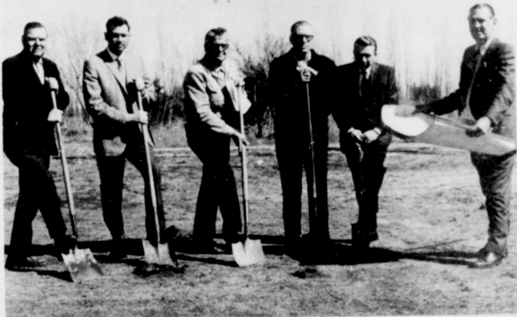
BREAK GROUND. . . Officials of the charitable trust corporation and the contractor for the 60 apartment units are shown as ground was broken for the project last Thursday. From the left is H.K. (Pudge) Kendrick, Gary Brown, Doyle Hunnicutt, Andy Hurst, Charles Allen and Bud Reynolds, contractor.
