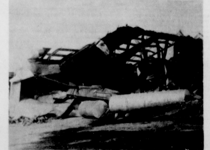
STORM FURY. . . This series of photographs, all taken on the Alton Morris place east of Lazbuddie, graphically illustrates the destruction brought about by the tornado which struck last Friday night. The Morris' brick home was demolished, killing Mrs. Morris. Another house and a steel barn were also wrecked along with trucks and farm implements.
