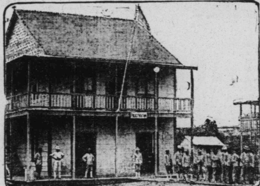
Here's the canal zone penitentiary and police station at Empire, thirty miles from Panama. The prisoners go out in chain gangs to cut weeds and grass and other things that harbor
