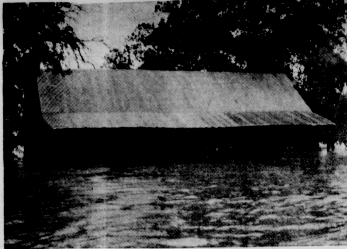
TWO EVACUATED—The J. W. "Pappy" Cox home in the West edge of Cross Plains was one of several flooded by a flash flood from Turkey Creek. This house, north of State Highway 36, contained about four or five feet of water. The picture was taken from a boat, owned by Edward Pancake, which evacuated two occupants of the house from higher ground West of the house. (Photo by Joe McNeel, Cross Plains Review)
