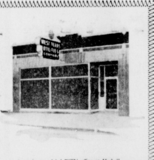
Recently remodeled WTU office at Haskell
