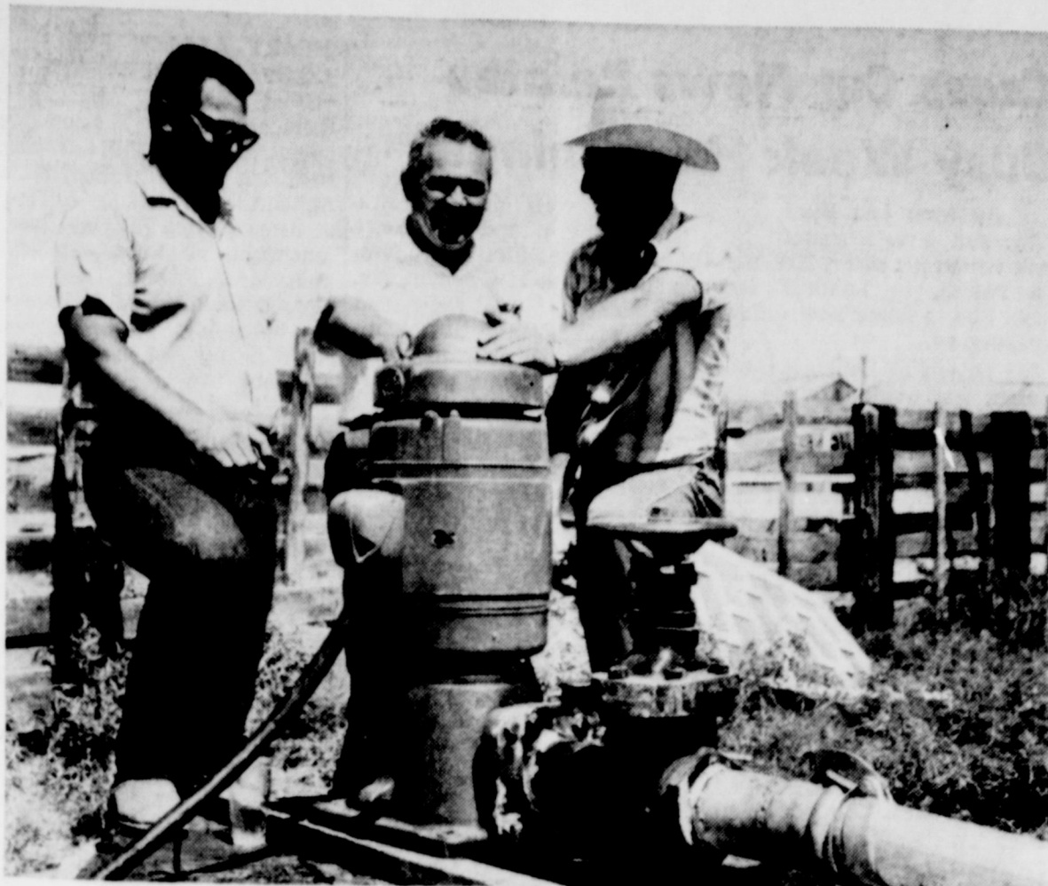
IT TAKES A BIG 'UN — Jack Leonard of Abilene and Woody Woodall of Lubbock stop to chat with Horace King about pumping equipment recently installed at his irrigation project in the Sabanno locality. King's wells are strong and require mechanization capable of handling a solid four-inch stream of water.
