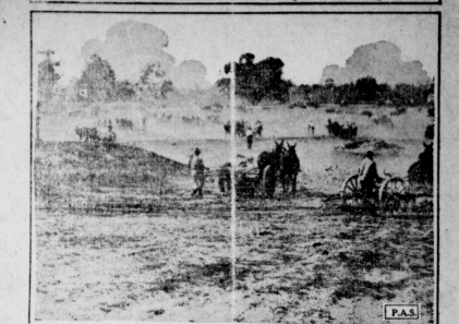
Ocala, Fla. . . Hundreds of mule-drawn scrapers are biting into Florida soil, digging the path which will be a sea-going canal across the state, joining the Gulf of Mexico with the Atlantic Ocean and thus taking coastwise ships out of the hurricane zone around the keys.
