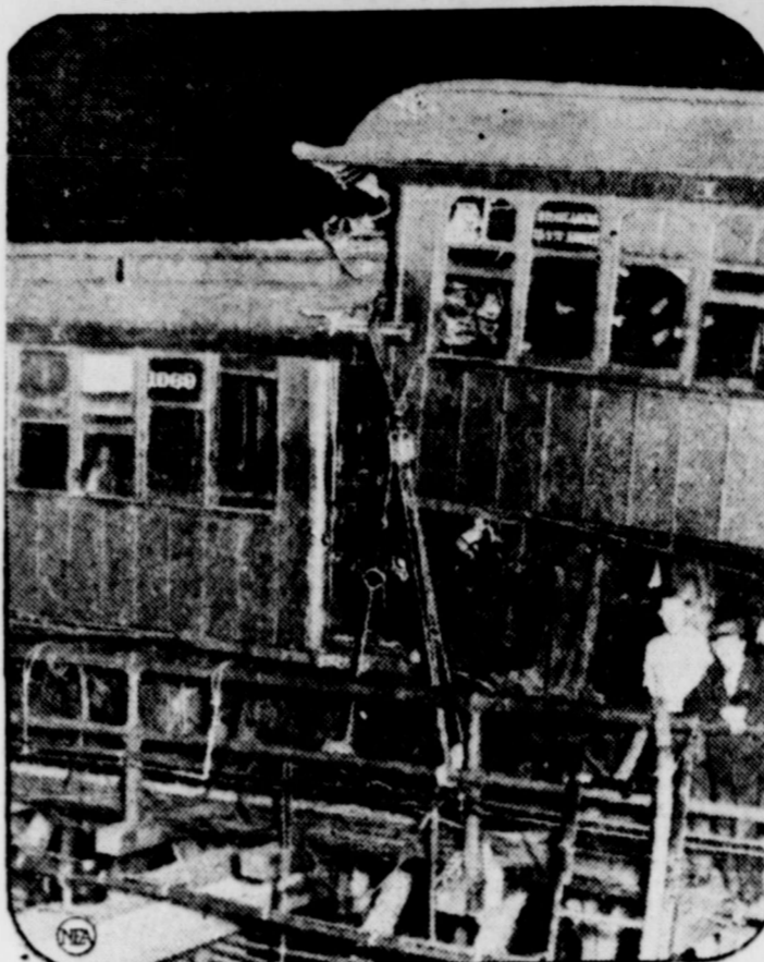
At the highest point on New York City's network of elevated lines—90 feet above the street—two passenger trains collided. Here you see the wreckage after one wooden train had telescoped the other, killing a guard and injuring 34 passengers. None of the cars toppled from the high structure, but the debris caught fire after the crash, causing a panic among passengers.
