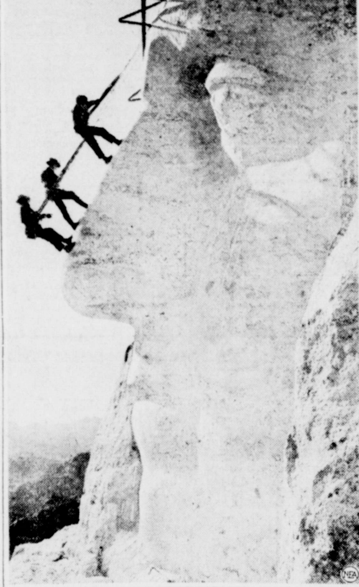
Carved in granite, the great stone face of George Washington is shown here looking down from the Mount Rushmore Memorial in the Black Hills of South Dakota. Size of the head, now nearing completion, is indicated by the men working on the nose. The head is 60 feet from chin to top of forehead and is built on the scale of a man 465 feet tall. Likenesses of Jefferson, Lincoln and Roosevelt also are being chiseled into the stone.
