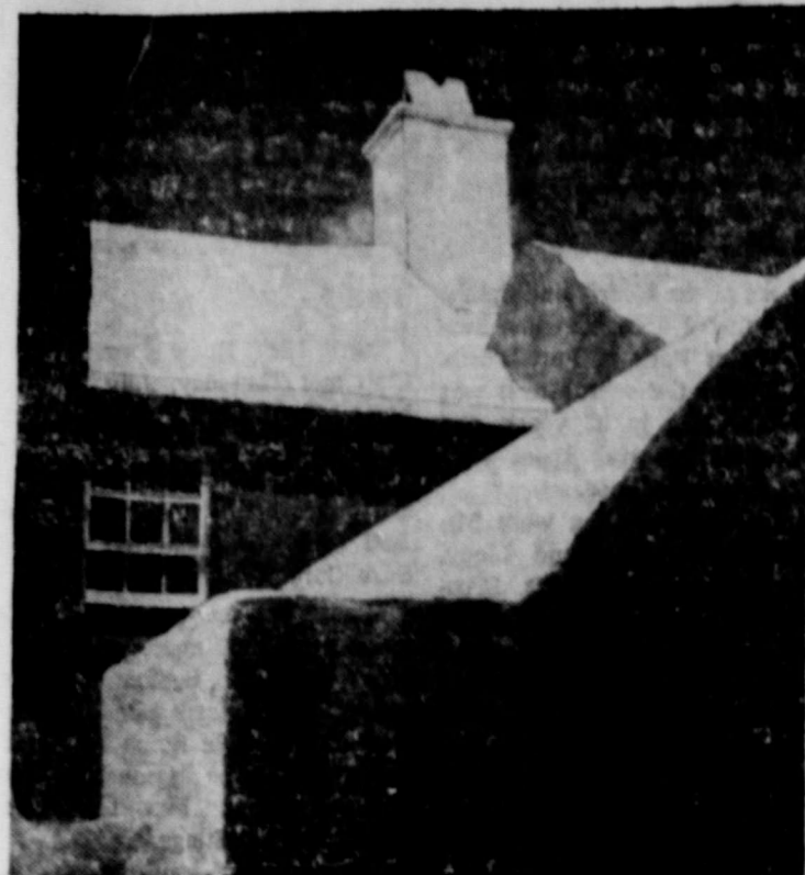
EARLY BERMUDA ARCHITECTURE: The years are kind to Bermuda's earliest homes, as sharper lines soften and blend into the quiet shadows such as "Frith's Cottage", built circa, 1705. The weird geometrical shape in the foreground is part of a water catch. The island has no natural water supply, so Bermudians must rely on the natural rain fall. Flutings line the white, coral slated roofs and lead to a water tank beneath the houses. F.N.S.
