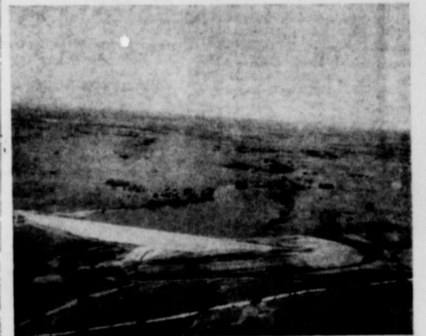
FLOOD PREVENTER—Site 24 on the B. J. Pruett and Henry Mayfield farms west of Hico is shown here following a 3.5 inch rain in late March. The structure detained runoff water, and released it slowly through the
