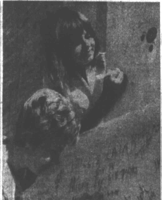
AUTOGRAPH, PLEASE—Debbie Woodard, top, and Phyllis Laird autograph a huge steel beam which will be used to "top out" the new Southwestern Bell Telephone Co. building under construction in Downtown Midland. Bell officials invite Midlanders to autograph the beam at the corner of Missouri and Marienfeld Streets prior to a "topping out" ceremony at 10 a.m. June 14. When the beam is attached, the building, although containing only seven stories, will be as tall as a normal 12-story structure.
