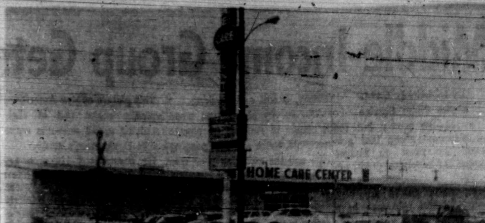
IN NEW HOME —The National Building Center, 3111 W. Front St., is spending its first Christmas season in the building recently completed next door to the old. A complete line of building and home care items can be found in NBC's Home Care Center and Don Bartley, manager, and his staff extend a warm invitation to the public to come by and look over the many gift items available.
