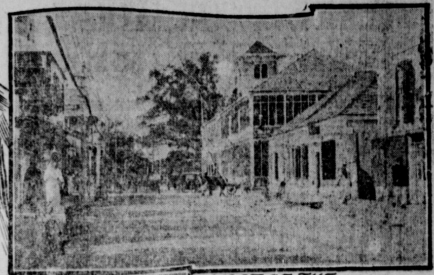
MOST OF THE BUILDINGS ARE WHITE
