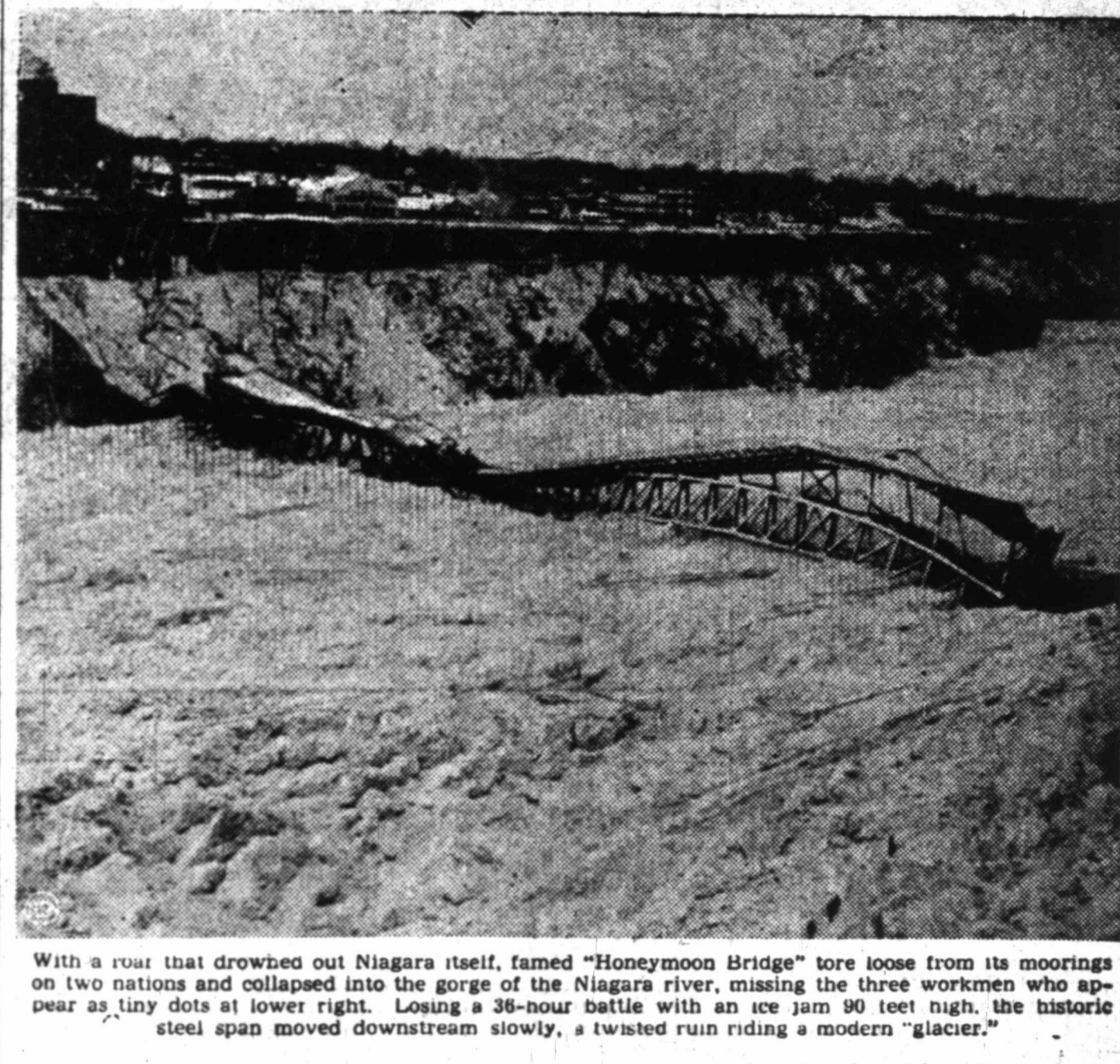
With a roar that drowned out Niagara itself, famed "Honeymoon Bridge" tore loose from its moorings on two nations and collapsed into the gorge of the Niagara river, missing the three workmen who appear as tiny dots at lower right. Losing a 36-hour battle with an ice jam 90 feet high, the historic steel span moved downstream slowly, a twisted ruin riding a modern "glacier."
