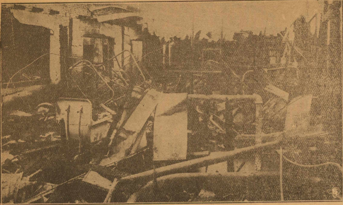
This picture of the De Soto Hotel, a small hostelry in Dallas' South Side, was taken immediately after firemen had rescued 25 guests without injury, and succeeded in getting the nine who were injured out with only one death resulting. The flames spread rapidly, after a beginning in the kitchen, and the hallways were turned into tunnels of flame, through which residents were forced to run to escape. Many jumped or climbed down firemen's ladders. J. E. Estill, 42, died of burns.
