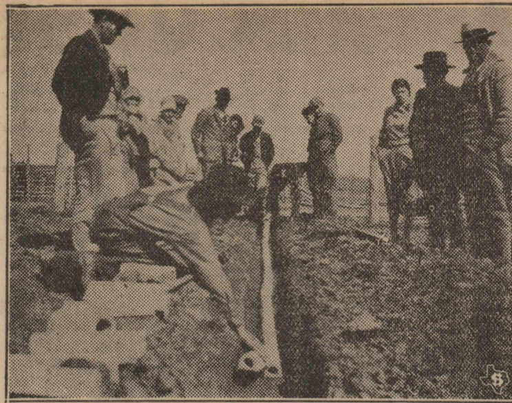
Here is shown a sub-irrigation installation in Grayson county, Texas, by B. F. Gray on the Hart farm. Sub-irrigating gardens using lath tile costing about one cent a foot is one of the big developments in gardening in Texas. The move is so strong this year that many are making cheap concrete tiles at home for the purpose.
