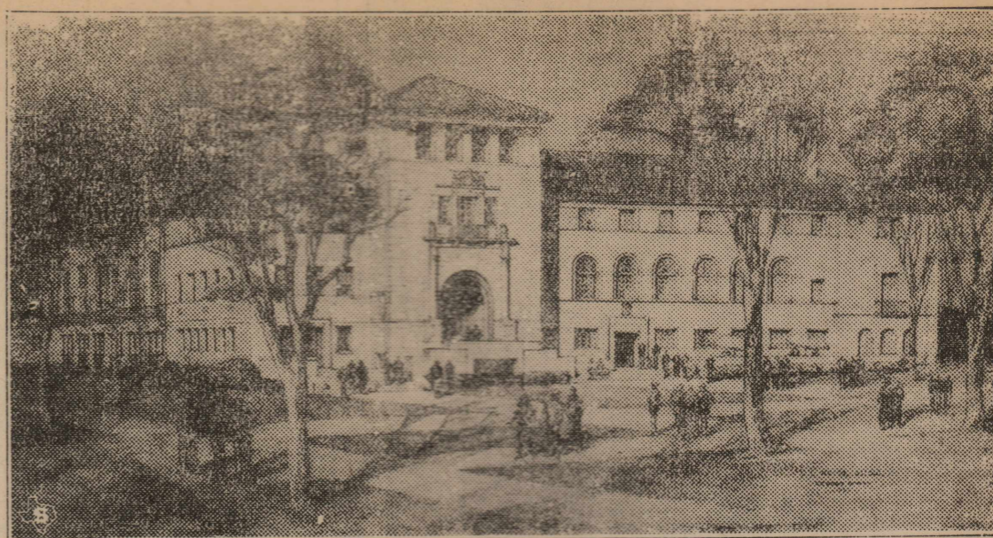
Here is the Union Building, one of the group of nine new buildings now under construction on the campus of Texas University at Austin. This building will be a student club building, social and recreational center. Nearly $3,500,000 is being expended in this gigantic building program.
