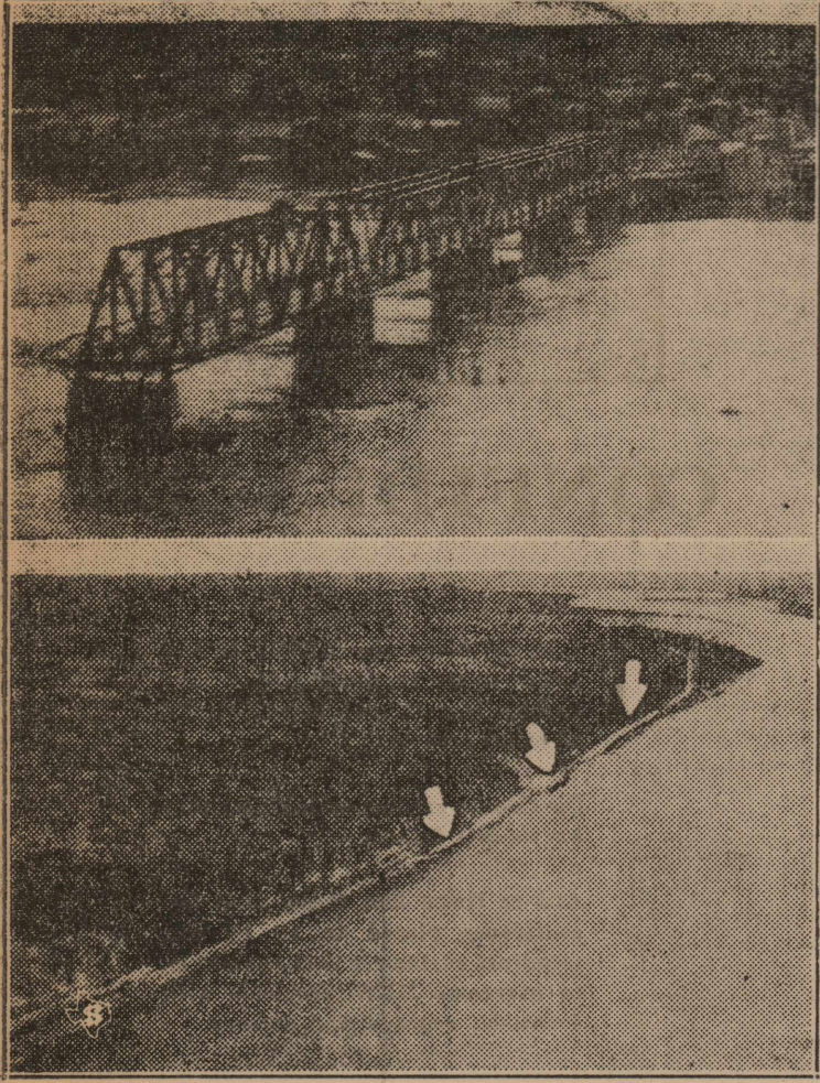
The top photo is a closeup aerial photo of the bridge over the Rio Grande river showing how the middle spans were washed away by debris piling up against them as the muddy waters swept towards the sea. Below is a section of the Southern Pacific tracks near Del Rio, inundated by the Rio Grande.
