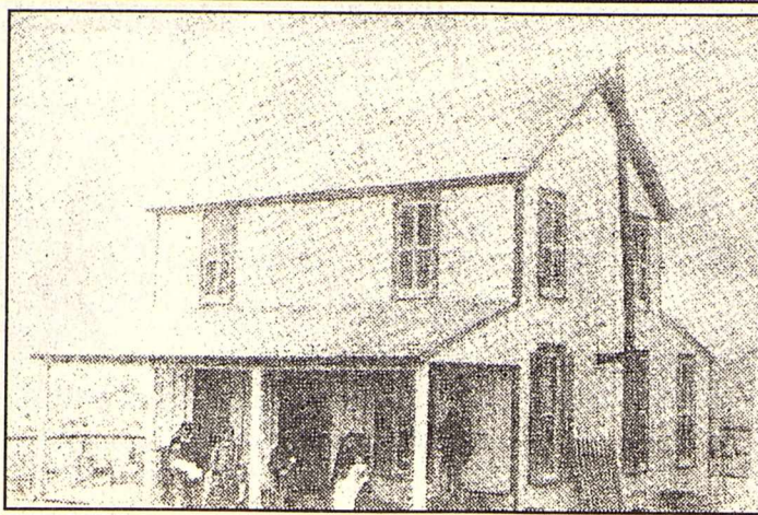
First meeting of the Commissioners Court of Sutton County was held December 1, 1890, in this house, the G.W. Morris home, the fifth house built in Sonora. The house was located on the east side of the present site of the Courthouse.
